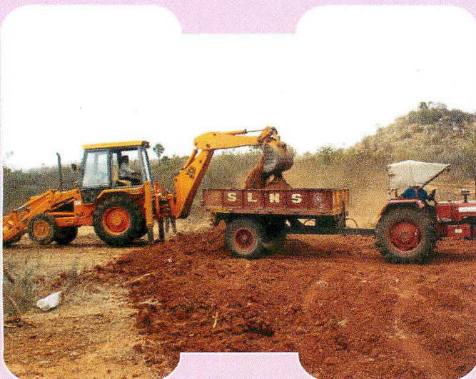
Development works in progress at Sector-V of East City
