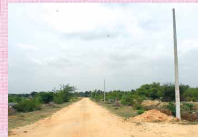
Electrical Poles at Sector - V
