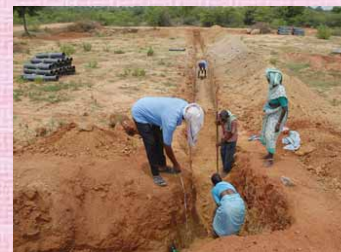
Sewage works Sector - V
